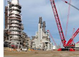
Crawler cranes <300t
